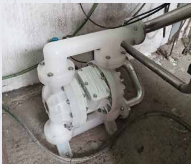
High fluid viscosity reduces pump delivery.
